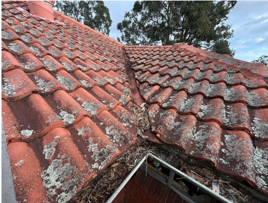
Existing valley iron to be replaced
